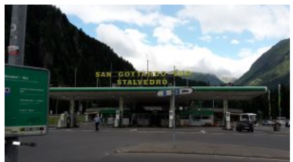
South Gotthard service station
